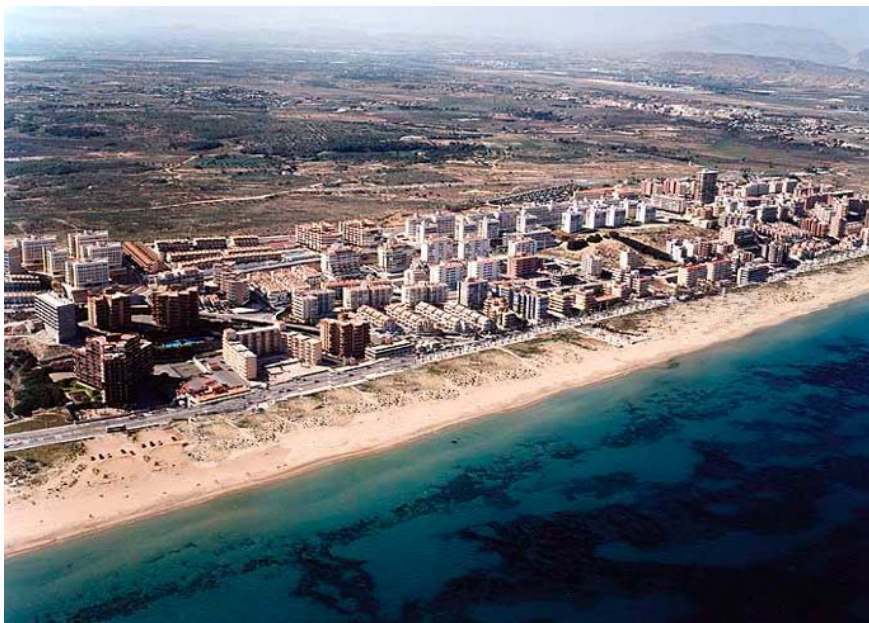
Figure 15: Simulation after the elimination of the buildings (Source: Environment Ministry)
