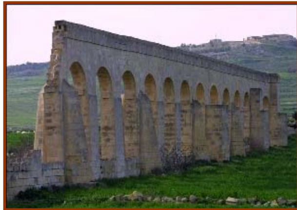
Remains of aquaduct on road to Gharb from Victoria
