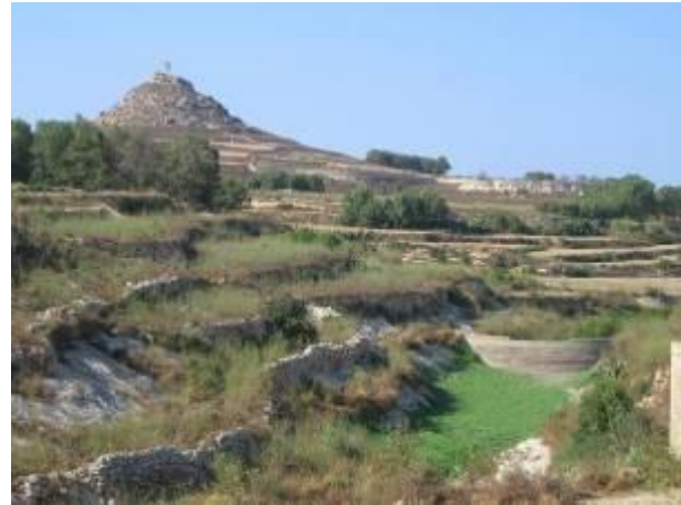
Fig. 15 Small dams are built to increase infiltration
