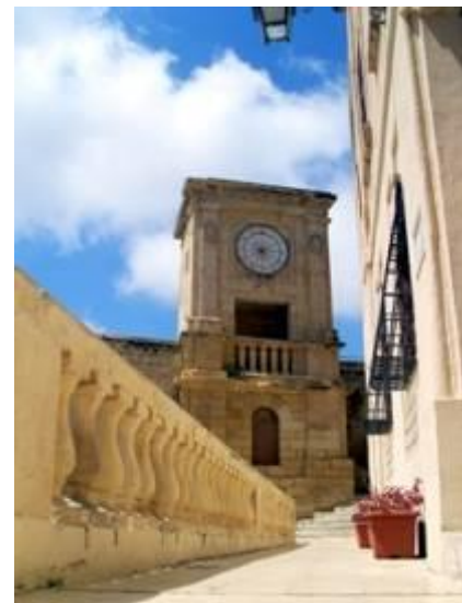
Fig. 3 Inside the Old Citadel
