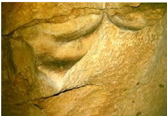
Fig.7: Corrosion notch, First Chamber, Level II.
