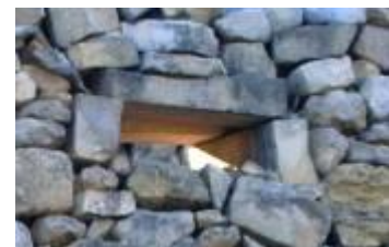
Fig.7: Detail of flow hole (Wied Qirda, Malta).
