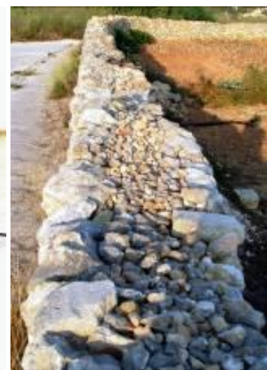
Fig.5: Rubble wall infill, ' mazkan ' (Wied Għomor, Malta).
