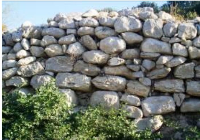
Fig.2: Rubble walls are 'dry' stone walls (Wied Qirda, Malta).
