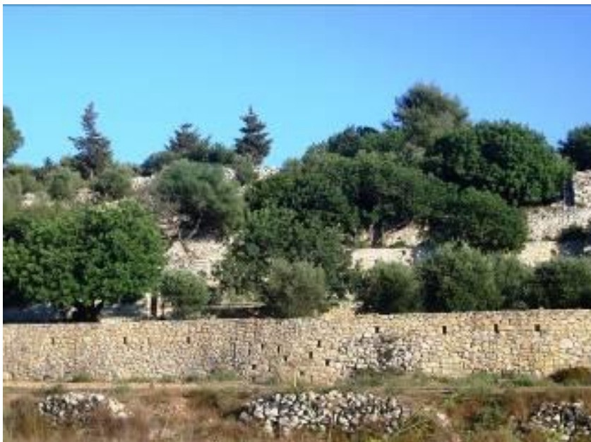
Fig.6: Flow holes in a rubble wall (Wied Qirda, Malta).
