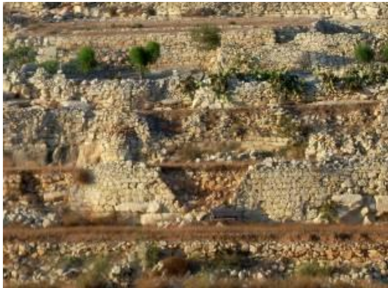
Fig.8: Rubble walls made up of ‘ Posta ’ and ‘ Ġwienaf ’ (Wied il-Kbir, Malta).
